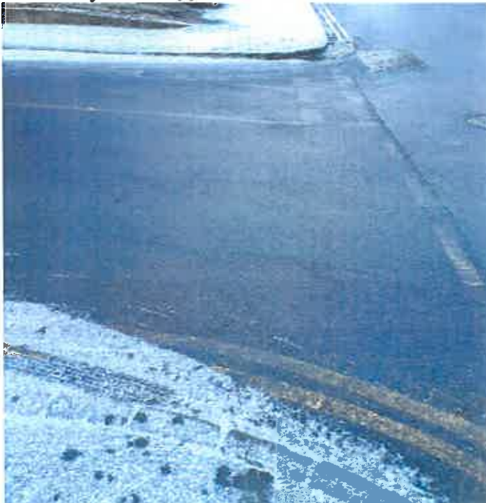
Figure 1 – junction of Harcourt Road and Framfield Road
