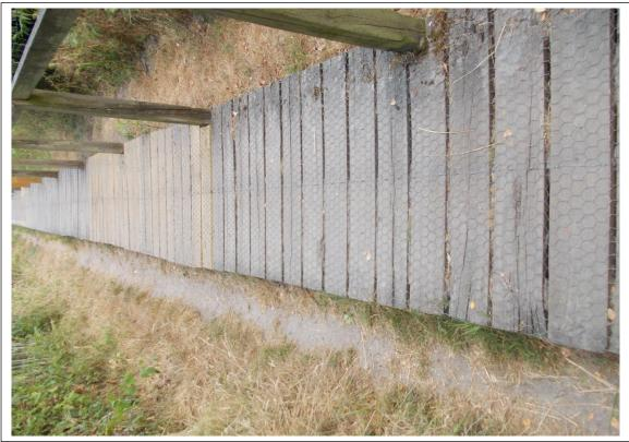
In the first year or so of maintenance much of the repair work involved replacing individual boards that have broken down. These are prised out once the netting has been peeled back and replaced before the netting is safely secured and usually several such could be done in a day on site. More recently it is evident that a few of the upright posts have rotted at about ground level and these have been replaced.
