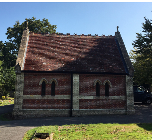
The Snatts Road Cemetery building was re-roofed using the existing tiles.
