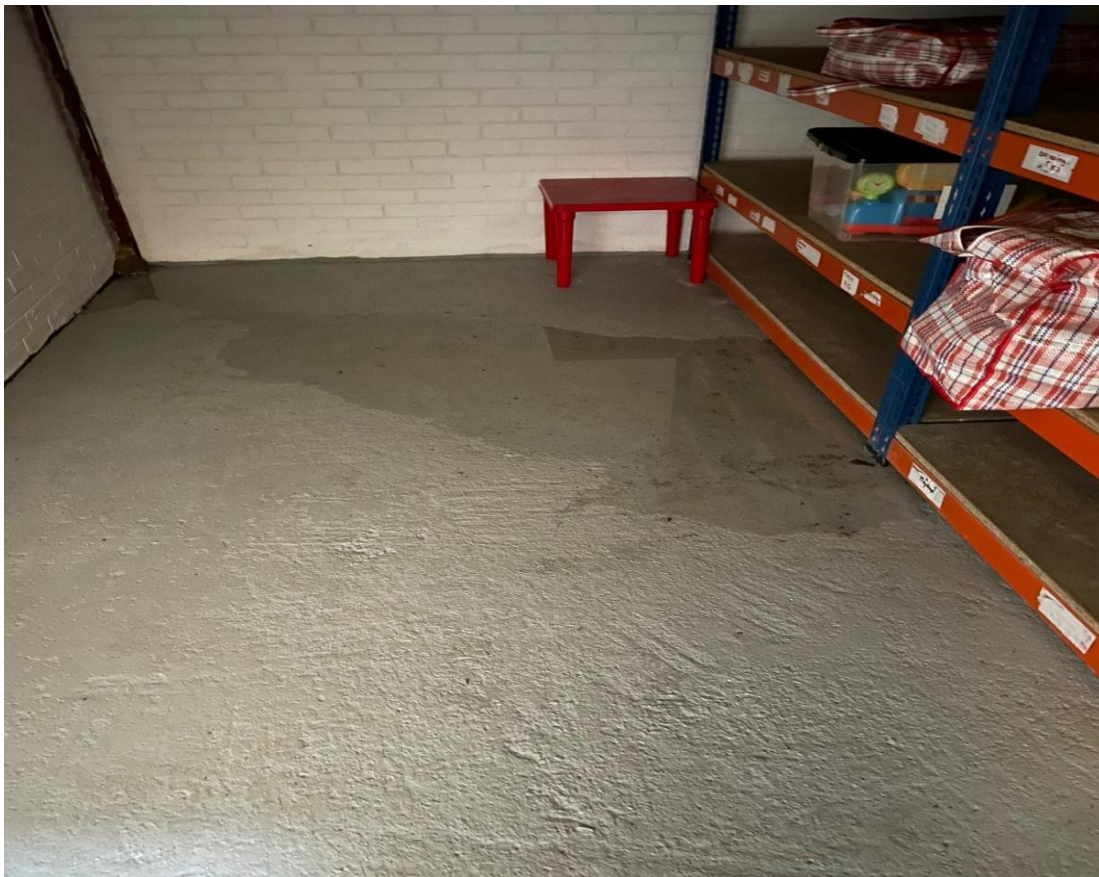
Figure 1: Front storage area (accessible from southern side of building)
