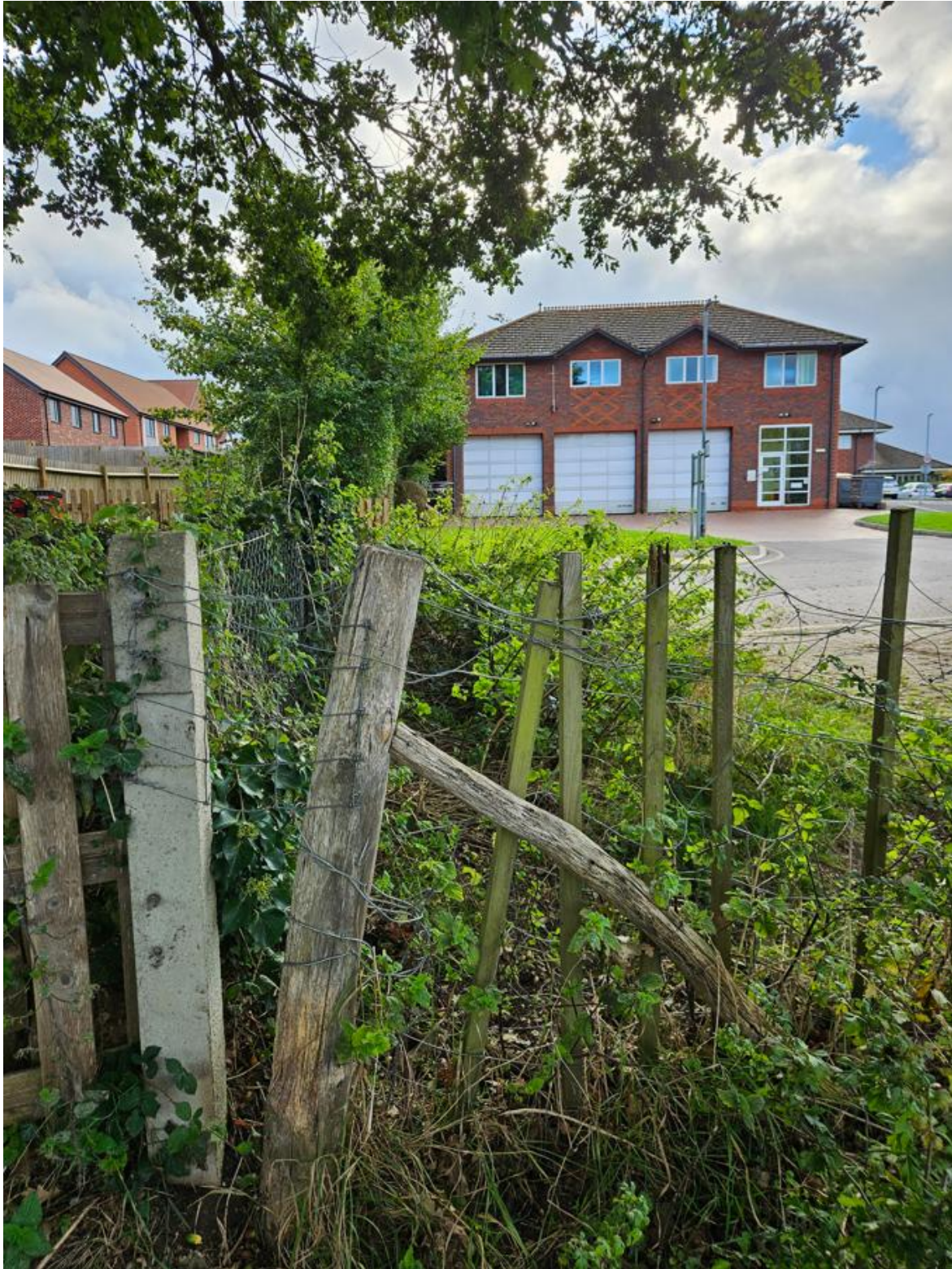
Image 4: Proposal for post to be re-installed to repair chain link fencing
